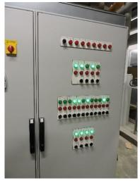
The buildings main heating, hot water and ventilation plant is controlled by a centralised building management system (BMS). This is controlled by a head end computer located in the facilities office.
