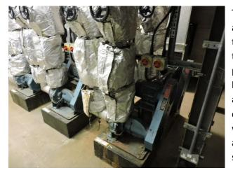
The existing heating and AHU motors and pumps within the building are, in the majority, fixed speed units meaning that they are either running at full power or they are off. In the training building these are VSD pumps running as a fixed 50Hz spend. In varying conditions the pumps and fan motors will only need to operate at part power and can consume less energy in doing so.
