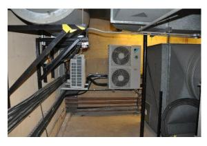
Within the Sports and Amenities (S&A) plant room there are number of split air conditioning units which are cooling sub server rooms and the UPS room. The external heat rejection elements of these systems have been located internally within the plant room which is itself a warm space and as these units are trying to reject heat they are having to work harder and consume more energy.
