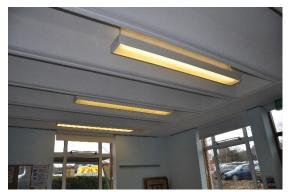
The lighting makes up a significant proportion of the electrical load across the site, and most areas are lit by a mixture of relatively efficient T5 fluorescent tubes, 2D fittings and some LED fittings as well as less efficient T8 fluorescent tube and PLL fittings.
