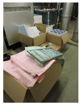
Filters in the supply air duct are necessary in order to remove any contaminants from the air being drawn into the building but they increase the resistance of the air flow and therefore increase the power used by VSD fan motors. The current filters are standard pleat and bag filters and are changed on a planned maintenance programme every 6 to 12 months.
