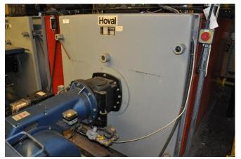
The boilers within both the S&A plant room and the Operations plant room are of a type which has a sectional burner unit. This sits on the front of the boiler and can be replaced independently of the boiler itself. The boiler casing and internal parts remain serviceable but the burner element where the combustion takes place is now inefficient and poorly controlled.
